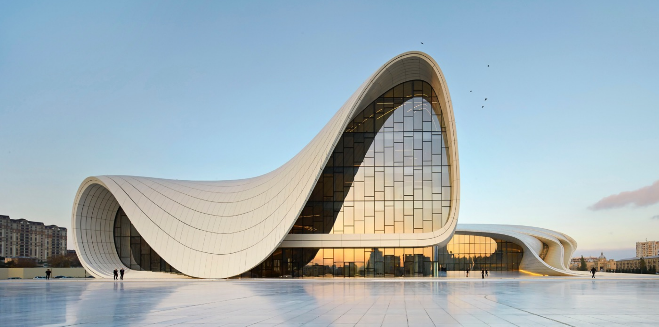
Heydar Aliyev Center, Zaha Hadid Architects
