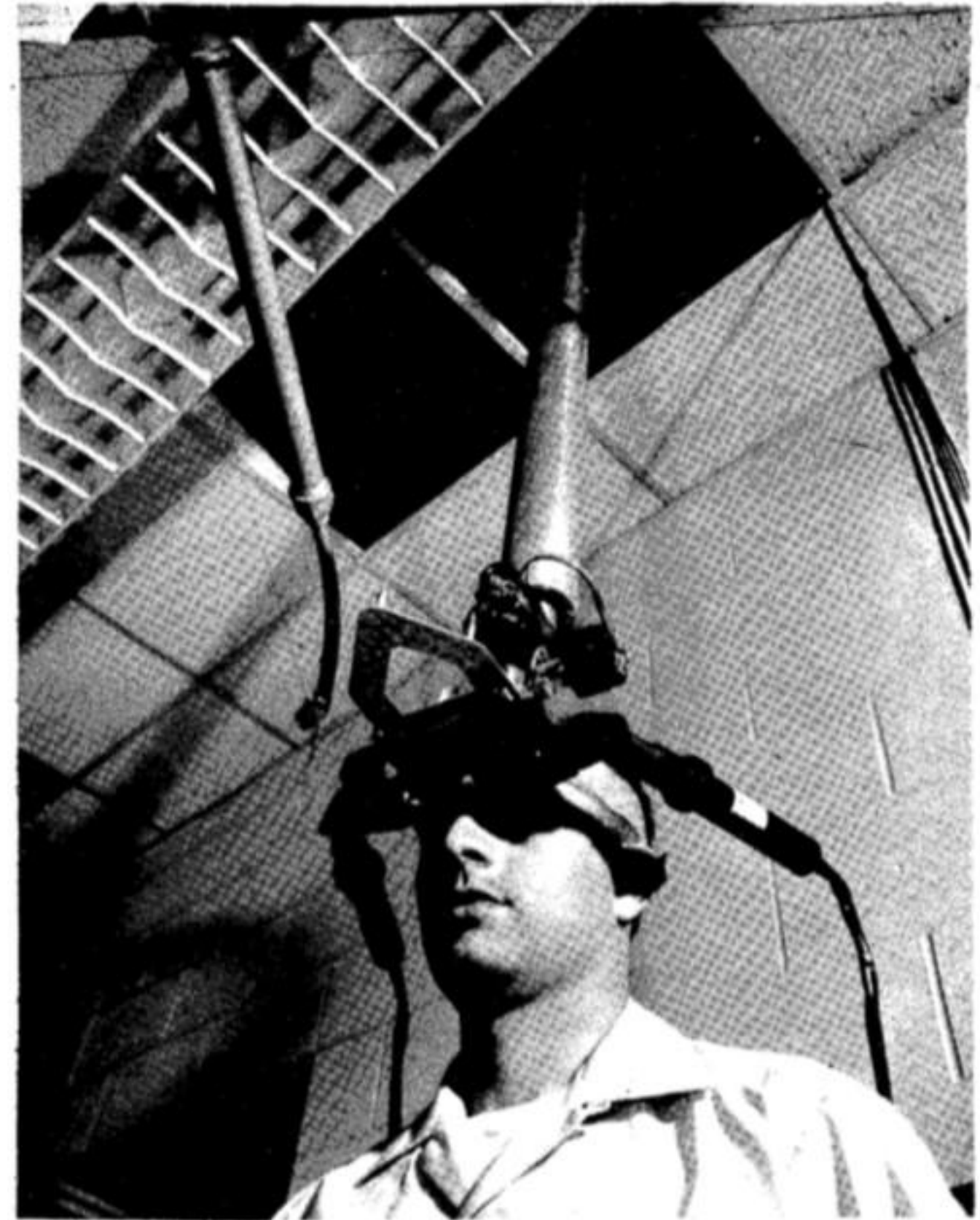
FIGURE 4—The ultrasonic head position sensor in use
